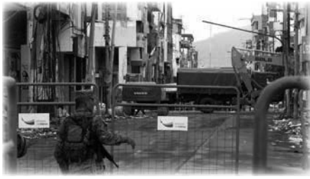
A Visit to Portoviejo in Ecuador Following the 2016 Earthquake
