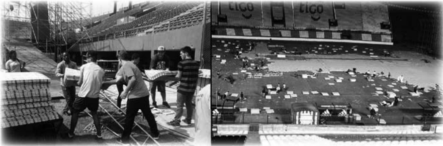
Laying the Temporary Pitch Covering for the Crusade in Paraguay
