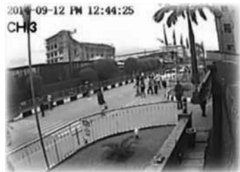
CCTV Footage Showing the Whole Building Collapsing Symmetrically
