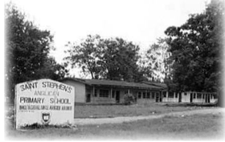
Saint Stephens lagere school in Arigidi
